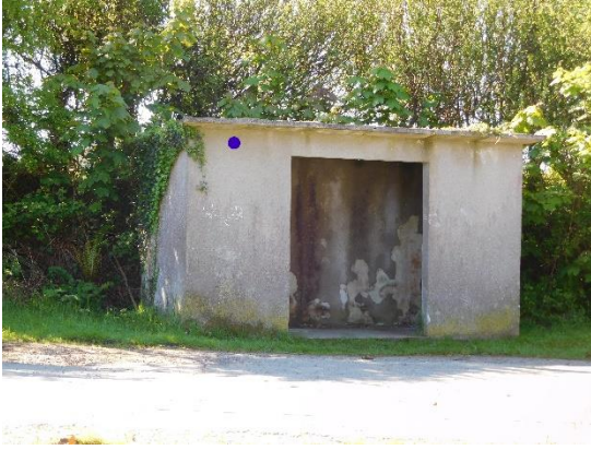
● Eniscaven Bus Shelter
